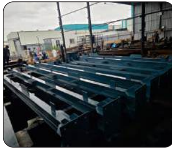
Boiler house structure
